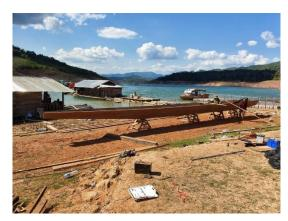
Construction was all steel nails and wooden pegs. The finish was a couple of coats of blue paint. Unfortunately, I did not get to see the finished boat in the water.
