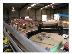
After partial deck removal, her engine was removed for reconditioning. Josh installed new flexible engine mounts, fuel tanks and skin fittings. Bolts were pulled and everything was stripped, checked and cleaned.
